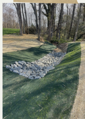
Lined Waterway & GSS
